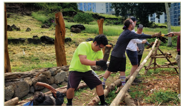
▲ We were honored to learn building techniques used by ancient Hawaiians to help build the foundation of a new hale.
