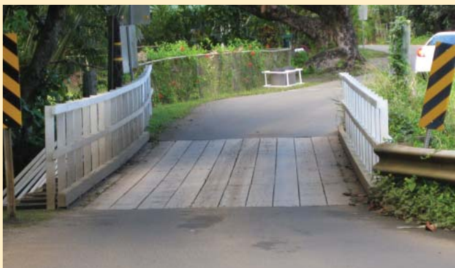
Old Wainiha Bridge No. 1.
