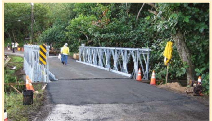
New Wainiha Bridge No. 1.
