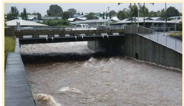
The flood channel in Kawaiilani Street Bridge during February 2008 flooding.
