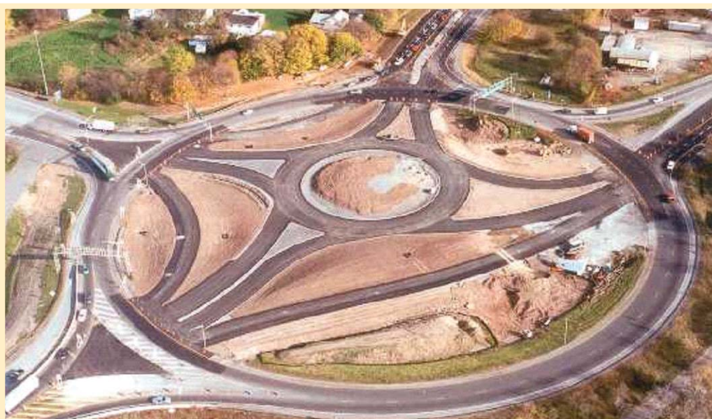
A New York rotary (outer circle) being replaced with a modern roundabout (inner circle) with bypass lanes. The newer design is expected to carry 10% more traffic than the prior design with fewer crashes. Photo NYDOT.
