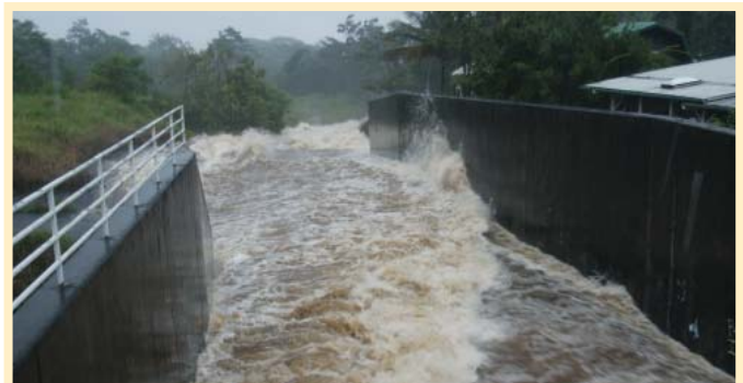
Komohana Street Bridge during February 2008 flooding.
