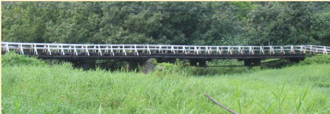
Old Wainiha Bridge No. 3.
