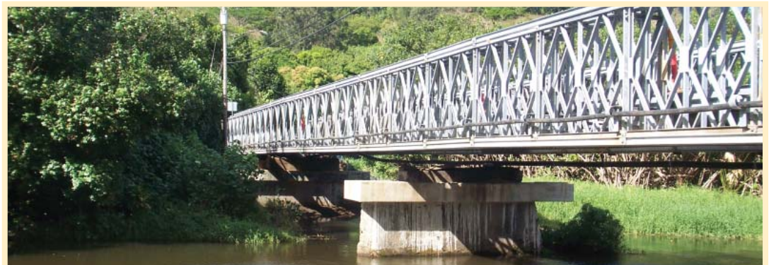
New Wainiha Bridge No. 3.
