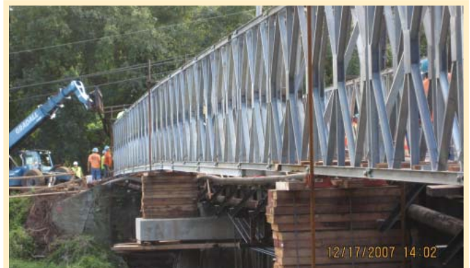
Wainiha Bridge No. 3 under construction.
